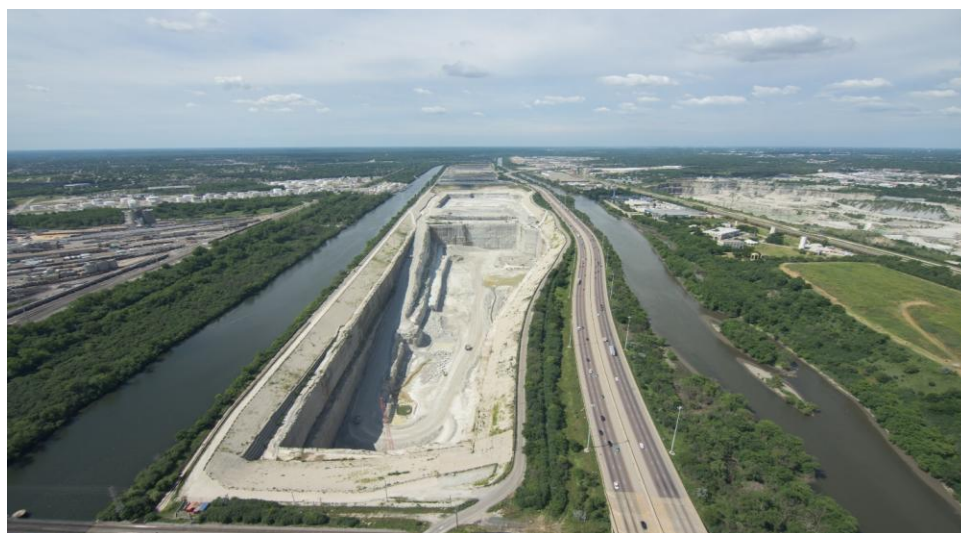
McCook Reservoir Stage 1, looking west. The Sanitary and Ship Canal is on the left, the Des Plaines River is on the right. MWRD Photo.
